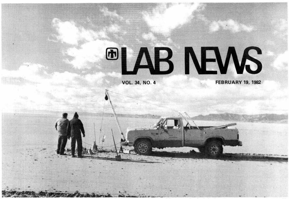
ON the barren mud flats that stretch forever in western Utah, two Sandia engineers examine their handiwork—the tail section of an earth penetrator dropped shortly before from a helicopter. The tail section detached from the penetrator and remained near the surface, by design, while the penetrator continued down some hundred-plus feet. Experiment is investigating possible use of penetrator for disposal of high level radwaste in ocean bottom sediment. Other photos, page four.
